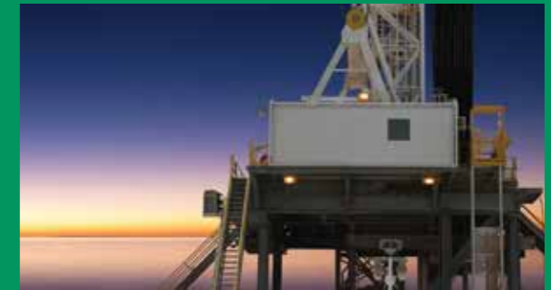
Control Unit for – Drilling Company
